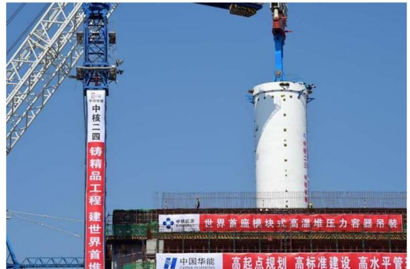
Figure 2. The pressure vessel of one of the HTGRs being installed at Huaneng Shidao Bay site in People's Republic of China in March 2016. China has signed memoranda of understanding with Saudi Arabia and United Arab Emirates for co-construction of HTGR nuclear power plants. Source: The State Council, People's Republic of China
